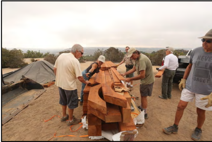
Construction on the Torrey Circle Pavilion Begins
