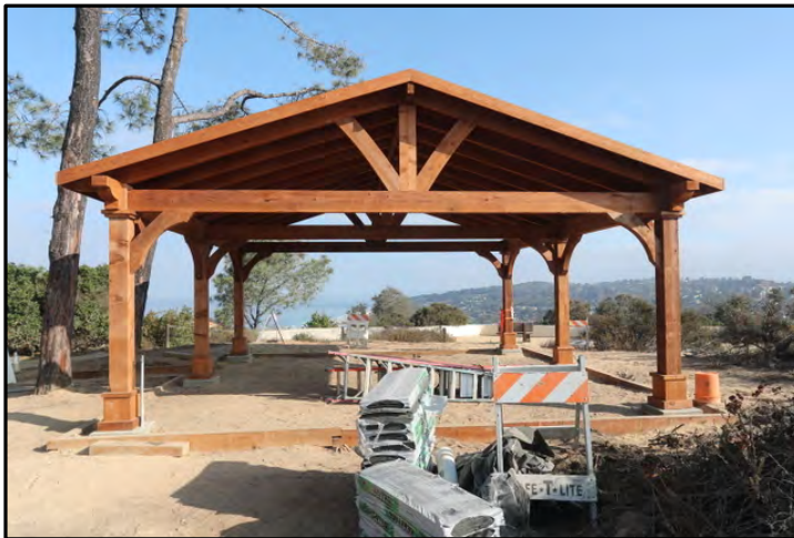
Great Progress as of August 25
