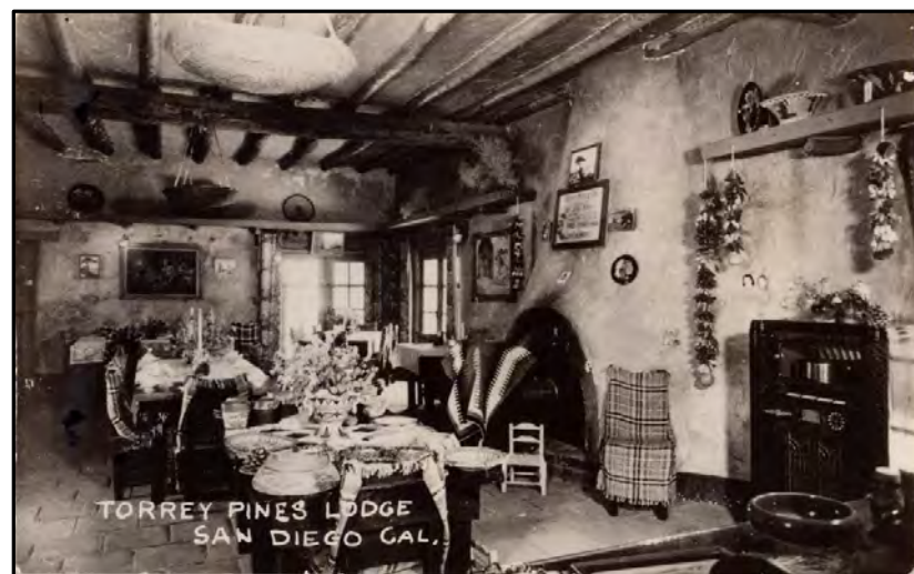
The inside of the Lodge, which was used as a restaurant from 1923. GIVE THE TOUR...lampshade, corner, fireplace, chile ristras; jukebox is from 1936/1937.
