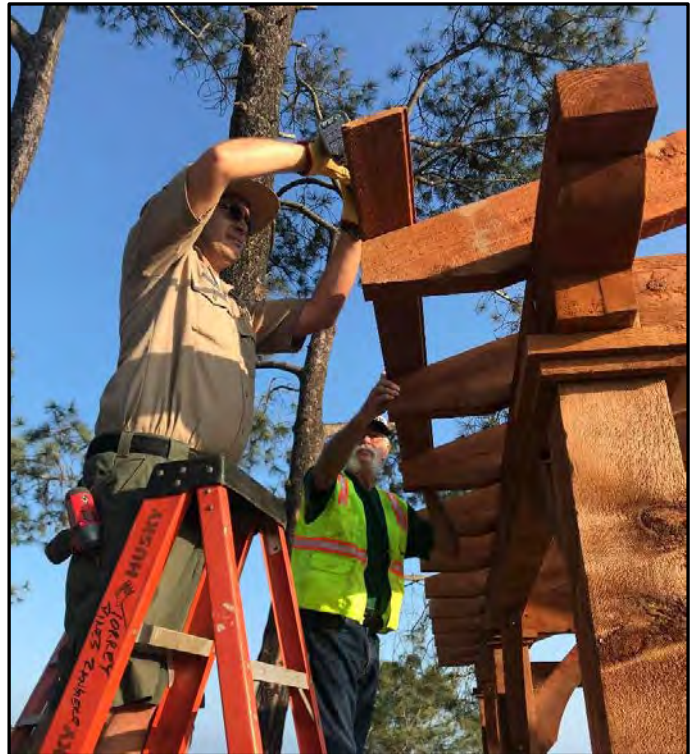
Dylan helping with the Pavilion assembly, August 2018
