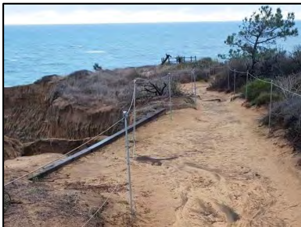
Razor Point Trail after repairs
