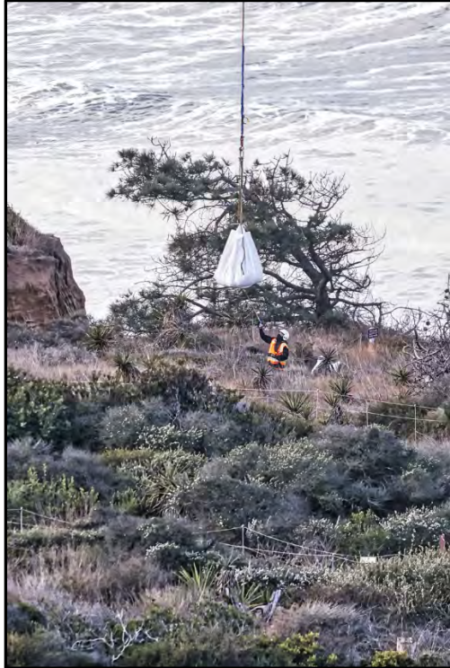
Helicopter dropping fill material; photo by Herb Knufken
