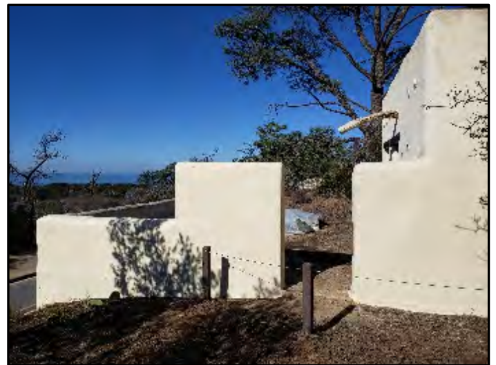
Lodge adobe wall after repairs
