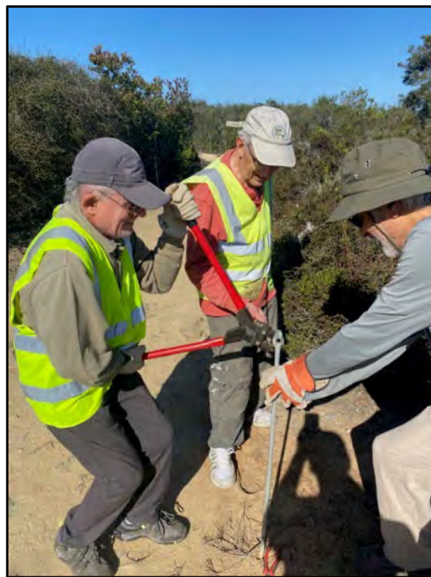
Thomas, Cliff, and Mukesh repairing eye-rod trail delineator damage Photo by Ingo Renner
