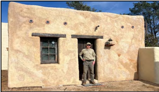
Corbin Schuppert in front of the re-plastered west wing of the Lodge
