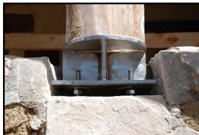
New inner column atop stainless-steel plate and concrete pier
