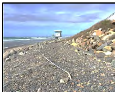
Note the handrail is almost completely covered by cobbles.
