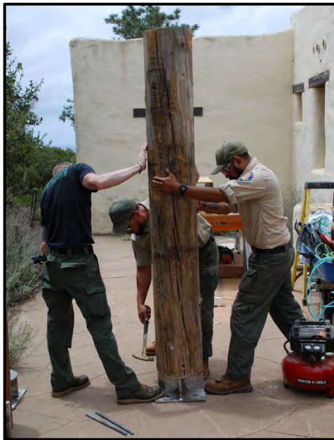
A new column being made; it fit perfectly.
