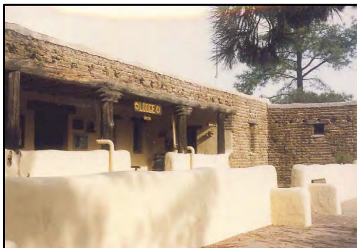
The front of Torrey Pines Lodge during a rehabilitation undertaken in 1986-87. Courtesy of California State Parks Southern Service Center Archival Collection.
