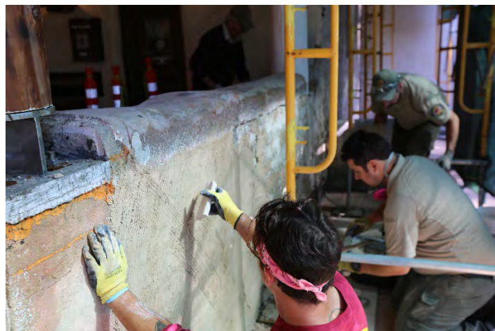
The Old Town maintenance team apply plaster and "scratch" it. Photo by John McCaull
