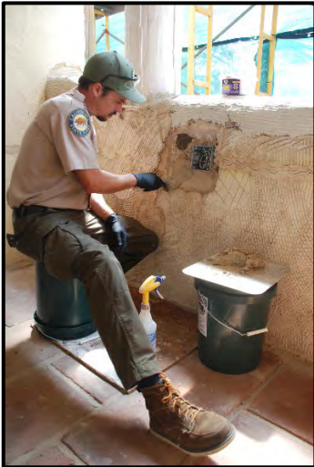
Torrey Pines maintenance aide Ryan Thiele shapes an angular mortared recess for restored porch lighting.
