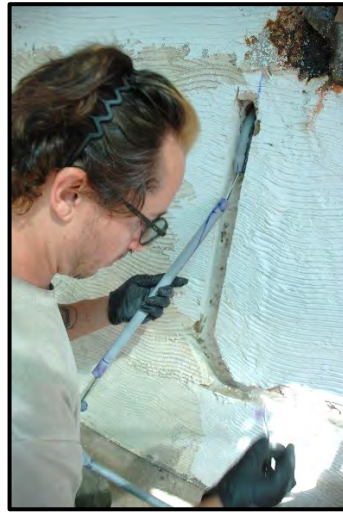
Old Town worker Wes Stoudor installs new electrical components within the adobe wall.
