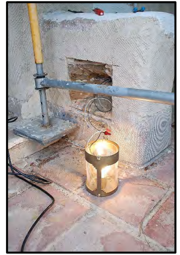
Testing the electricity: "We have light!"
