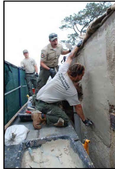
Wes Stoudor leads Old Town recruits through the “brown-coat” plastering stage.
