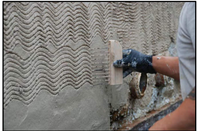
A tight, wavy “key” is made in the “brown-coat” with finesse and a plaster-comb.
