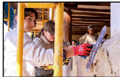
Rowan Jackman hard at work plastering Photo: Isaac Ullah, SDSU
